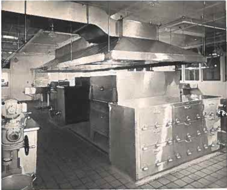
Main Kitchen, Plate No. 927
